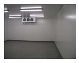
Sandwich-panels have three layer structure with thickness from 40 to 200 mm, consisting of two metal layers (or other sheet material) and a hard polyurethane core between them.
